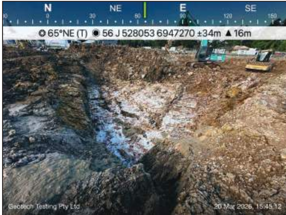
Photo 1: Removal of Wet/Soft Material
