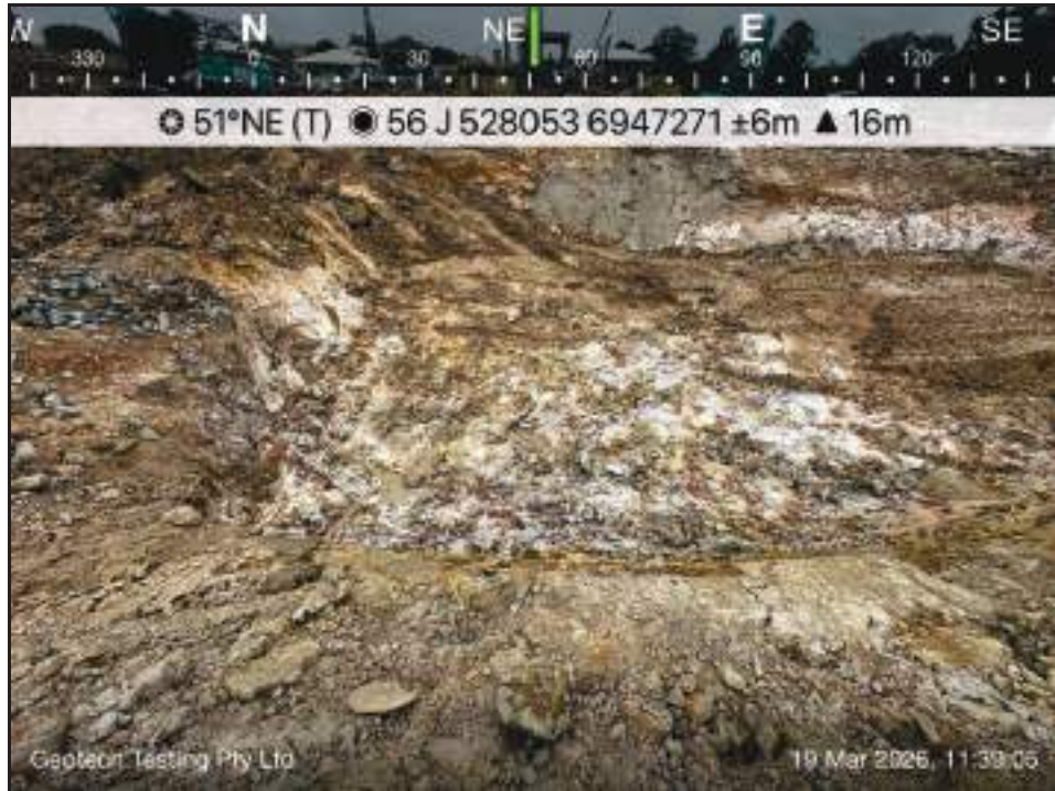
Photo 1: Removal of Wet/Soft Material
