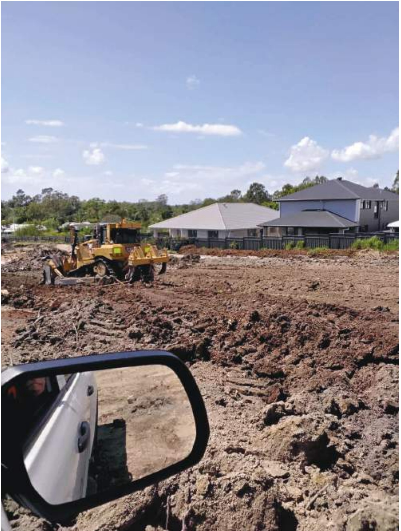
RIPPED SUB SURFACE
