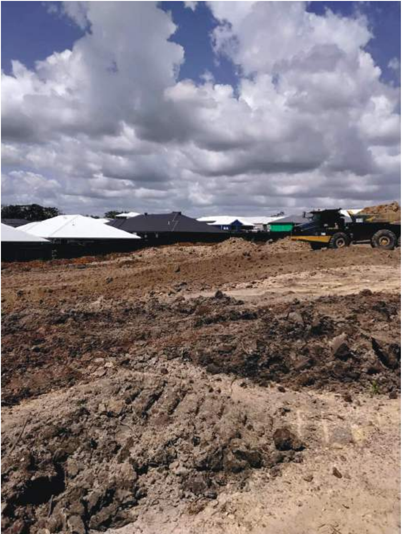
RIPPED SUB SURFACE
